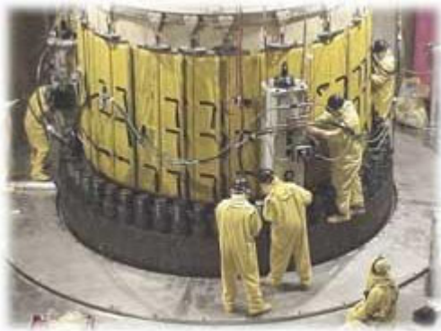
Tensioning reactor pressure vessel at SONGS
