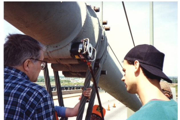
Below: Equipment being used on the Delaware Memorial Bridge
